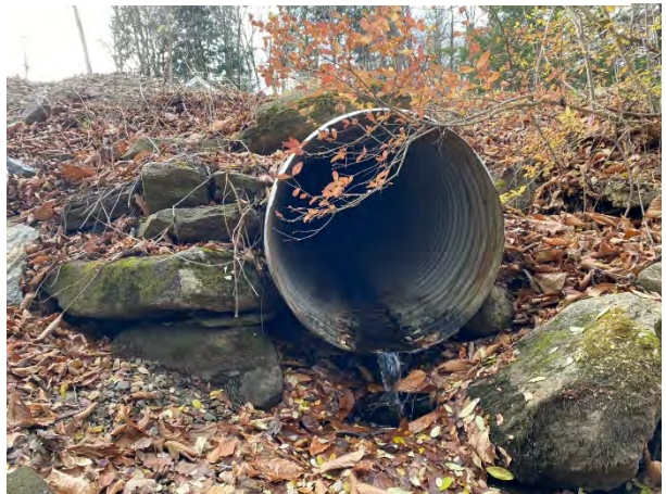
Figure A-6. Outlet pipe from cistern.
