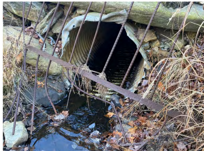
Figure A-13. Culvert inlet with debris grate.
