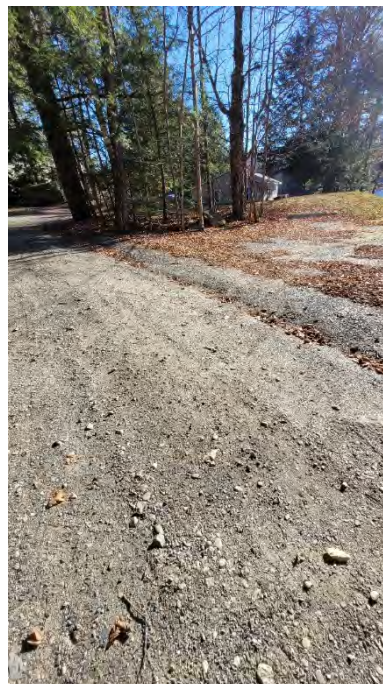
Figure A-31. Road erosion on Anderson Road and low area that floods adjacent lawns.
