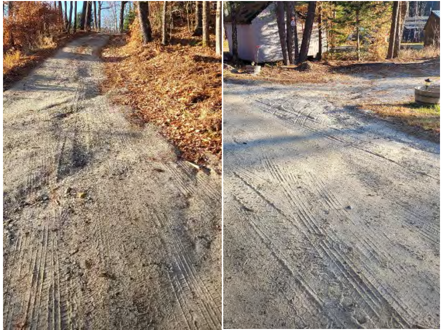
Figure A-10. Emerson Road erosion into driveway.
