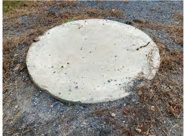
Figure A-5. Cistern structure that collects drainage pipes from around property.
