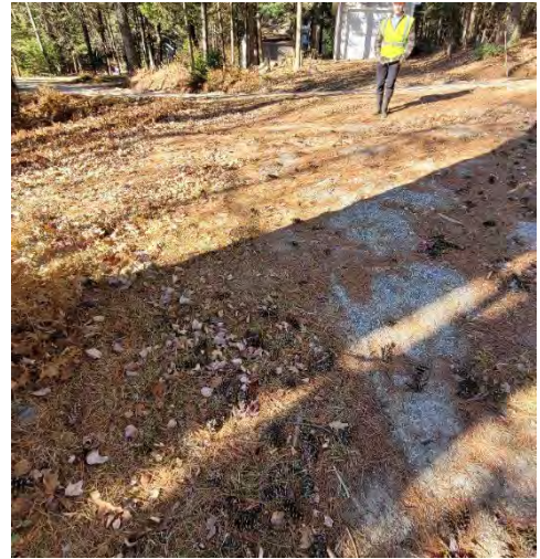
Figure A-17. Accumulated sediment on Shorewood Estates Road low point.
