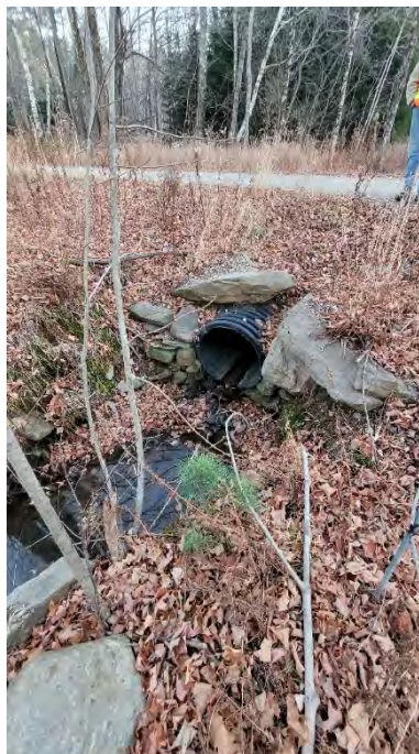
Figure A-25. Culvert crossing Gove Road and erosion downstream.
