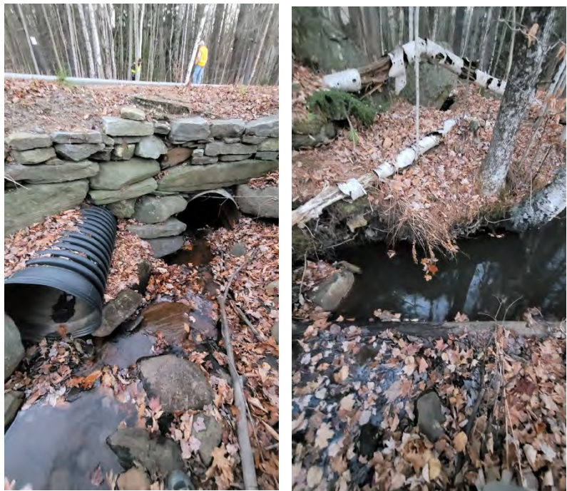
Figure A-27. Upstream culvert inlets and downstream bank scour.
