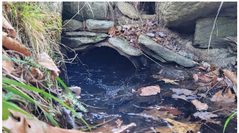
Figure A-34. Outlet of undersized culvert under Crescent Lake Road.
