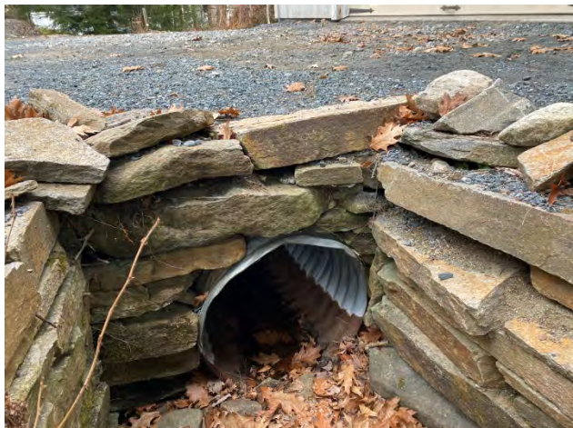
Figure A-9. 90 degree driveway culvert.
