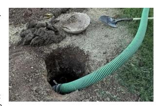
wastewater generated by the use of appliances such as dishwashers, washing machines, etc. should also be considered. The EPA recommends that a septic system should be pumped every three to five years and a full system inspection should be done every three years. NH DES recommends pumping every two to three years. A professional septic inspector can advise you of any irregularities in the system and need for repair.
